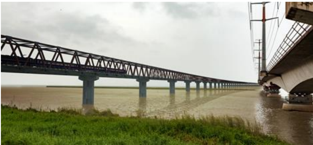
Figure 3. Bangabandhu Sheikh Mujib Railway Bridge Construction Project, Bangladesh (on-going)
